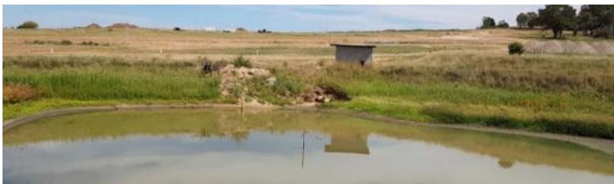
Plate 4 Farm dam no.5, facing west towards the abandoned pump house
